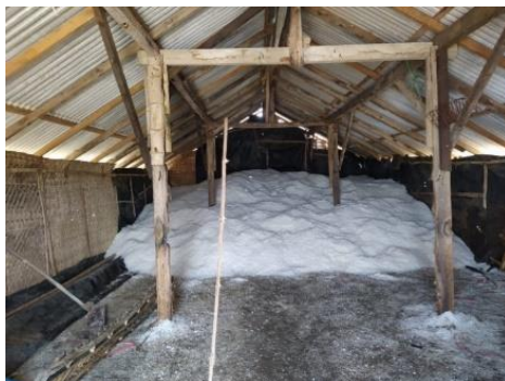
Figure 2. Salt Storage Warehouse
